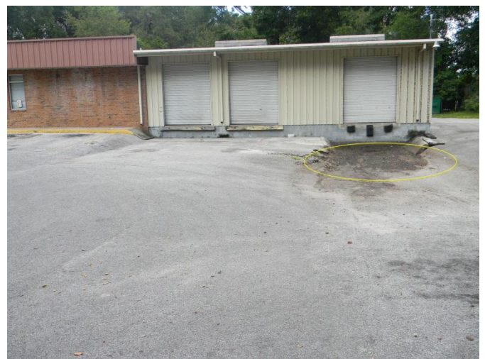
Example of deteriorating pavement
