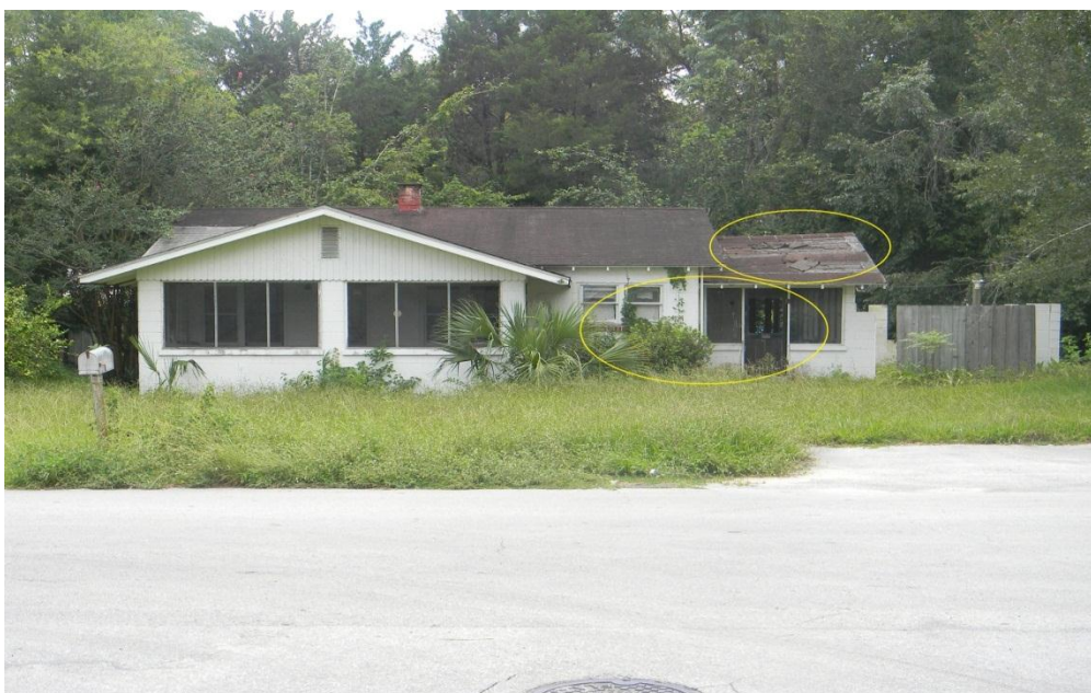
Example of deteriorating roof, walls,
