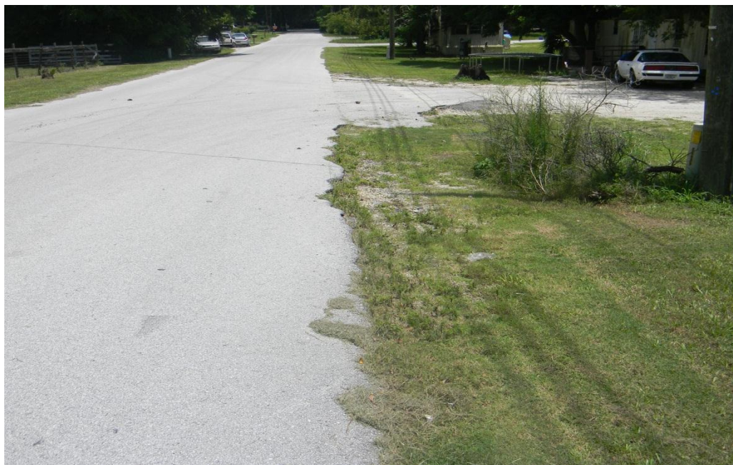
Example of broken / deteriorating roadway pavement
