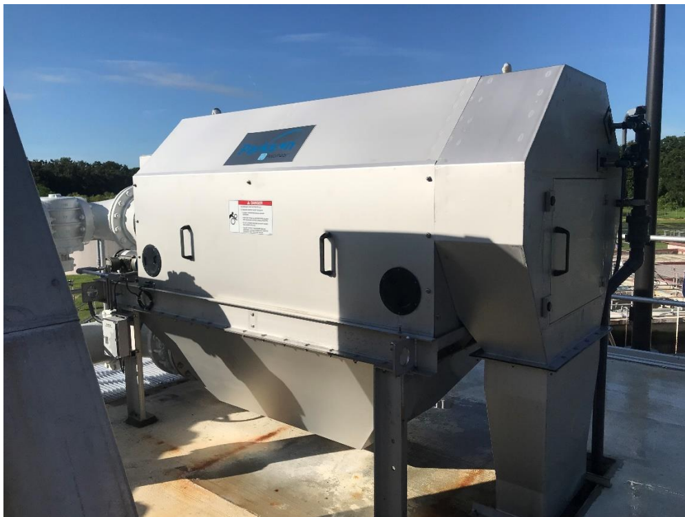
Figure 8. Existing Drum Screen
