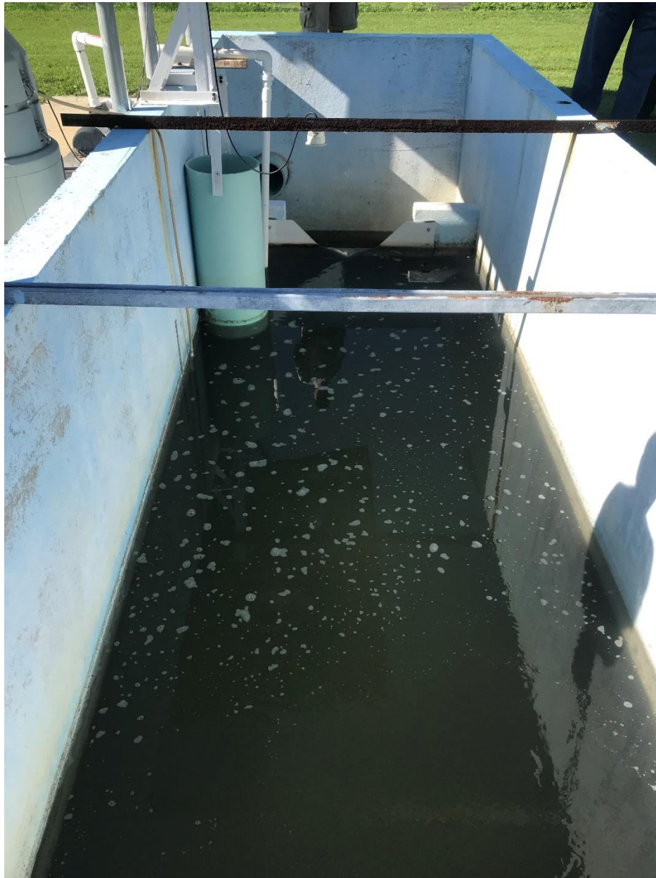
Figure 13. Effluent V-Notch Weir and Level Indicator
