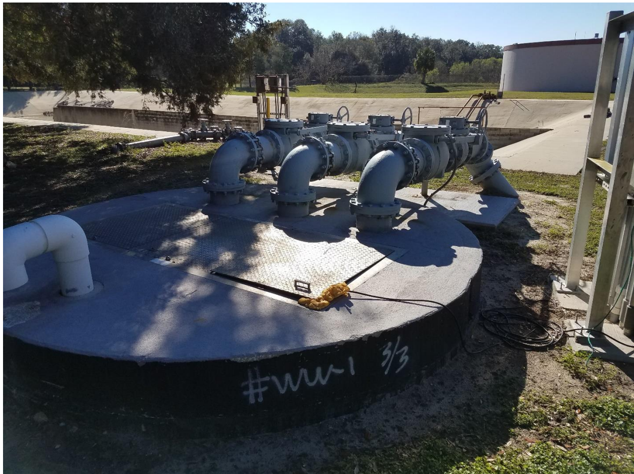
Figure 3. Influent lift station
